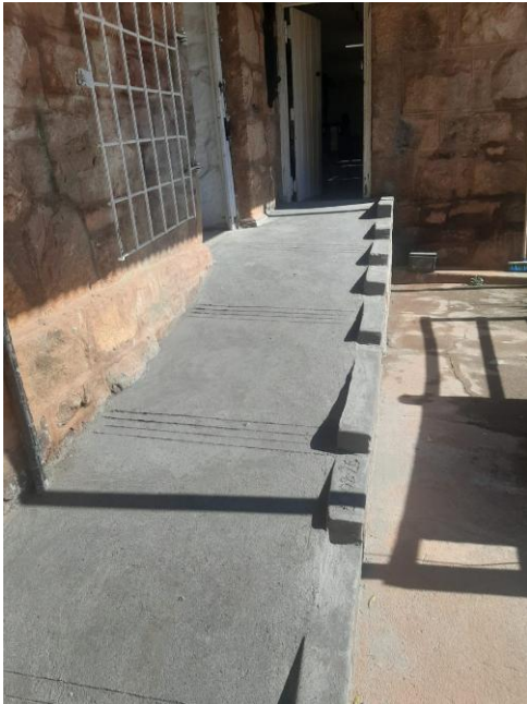
New wheelchair ramp
